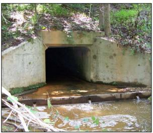
**Poorly-sized or Installed Culverts:** Undersized culverts restrict natural stream flows, particularly during floods. Water exits the structure at a high velocity, causing channel and bank erosion. Overly-wide culverts spread a stream's flow out over a wide area, so water depths are too shallow for many fish and other aquatic organisms to swim or move through.
